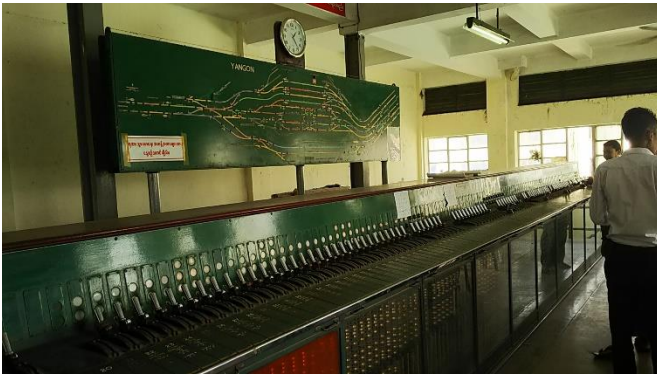
Ex-interlocking devices (manufactured in UK in 1941) Electronic interlocking devices (manufactured in Japan)
